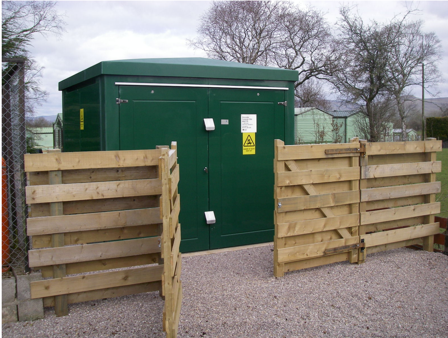
Substation (metal or plastic housing)
