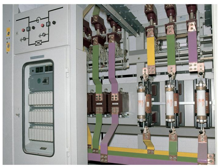
Is-limiter connected in parallel with a reactor – fixed mounted –
