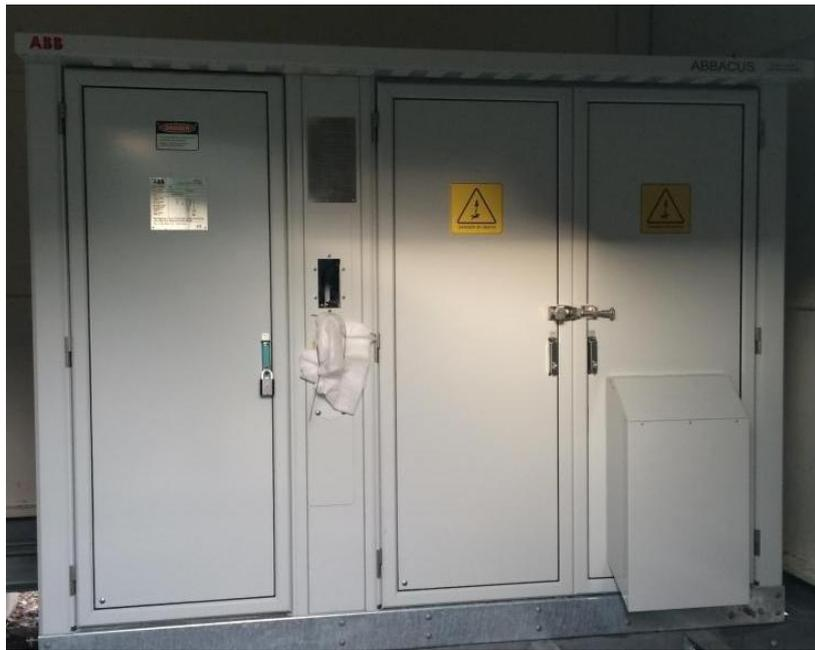
These capacitors are also controlled by the CQ930 RTU (Figure 7) that is used with the LV capacitor. The only difference in operation is that the HV capacitors do not use multi-stage switching. Each GM capacitor bank system comprises of one incoming stage and one switched power stage.
