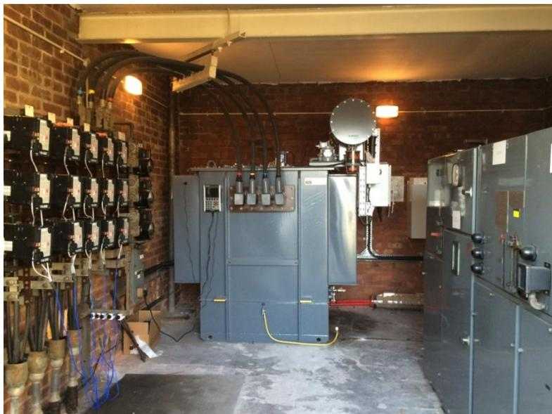
As part of Smart Street, Electricity North West has installed five distribution transformers with an on-load tap changer (Figure 11). These transformers are a standard distribution transformer with the addition of:
