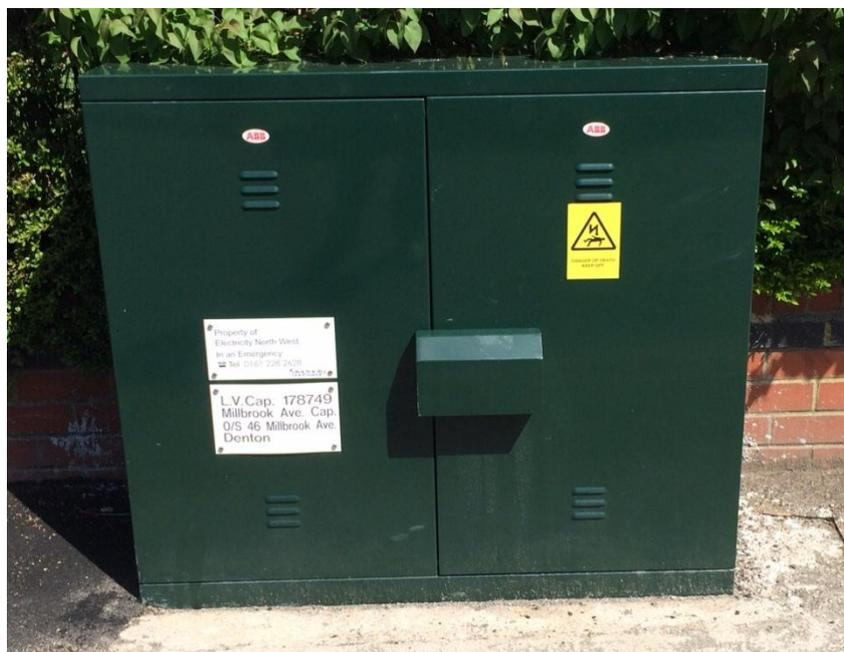
There are 84 LV capacitors (Figure 6) in total deployed on Smart Street trial circuits. These capacitors will provide a voltage boost at the point of connection; this allows the control system to optimise the voltage along the LV feeders depending on the load.
